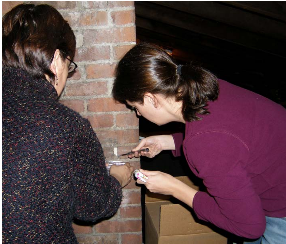
Kress Fellows in Historic Preservation removing mortar at the Bartow-Pell Mansion Museum, located in a historic house in New York City.
